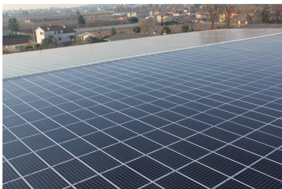
Italy: 1 MW 2661 monocrystalline modules of 260 Wp
