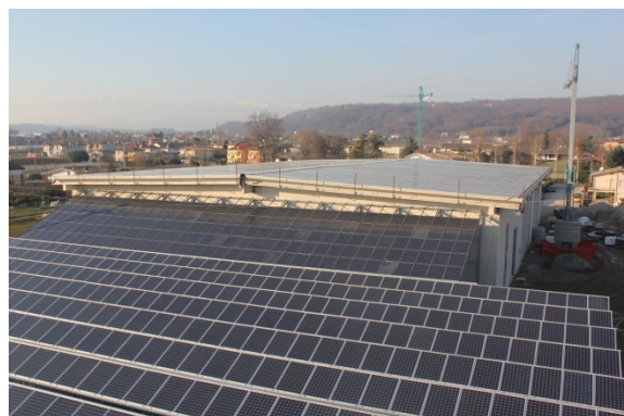
Italy: 1 MW 2661 monocrystalline modules of 260 Wp
