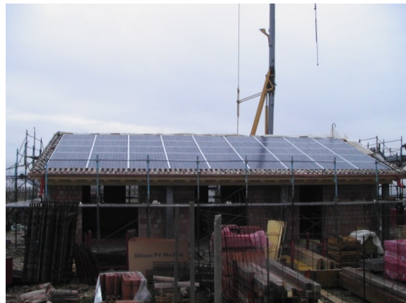
Italy: 12 kW 45 monocrystalline modules of 260 Wp
