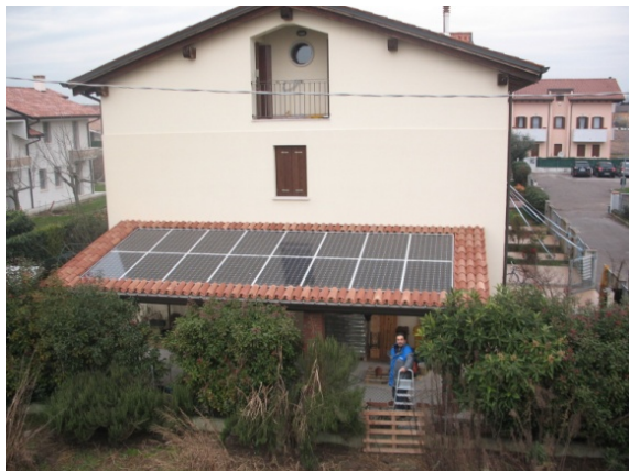
Italy: 4 kW 16 monocrystalline modules of 260 Wp
